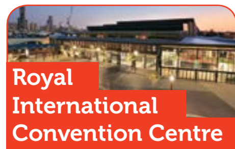
Royal International Convention Centre The state-of-the-art Royal ICC offers world-class service for conferences, major events, exhibitions, banquets and weddings within a boutique convention centre, just 1.5km from Brisbane's CBD.
