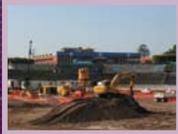
Bypass tunnel update
