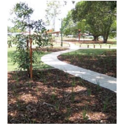
On location at the Nudgee State School revitalisation project
